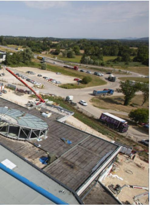
In this type of work situation, the risk of slipping and falling is higher. A safety device must be installed to guard against these hazards.
